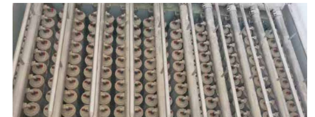
Rongcheng Water Plant, Xiong'an
